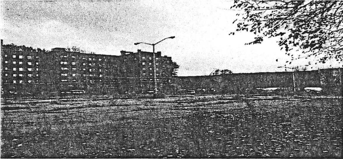
Location of Future Midrise Building
